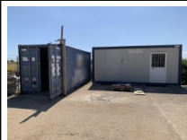
#21: Container and Office Box
